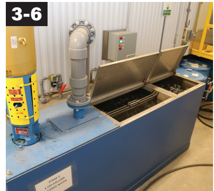
3-6 Clean: City water rinse Cleaner: Recycling reverse osmosis water rinse Cleanest: Pure reverse osmosis water rinse Sealer: Dried-in-place aluminum sealer
