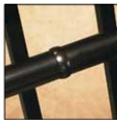
Collar Ring (to cover splice)
